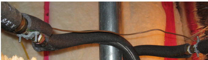
E3509.6 Metal water piping bonding.
