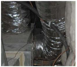
The flexible ducts rested on each other in some areas. Flexible ducts are not designed to support the weight
